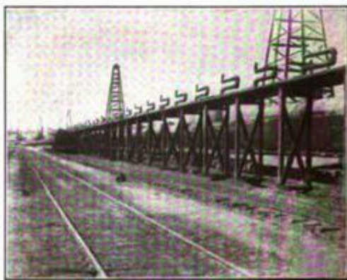
Loading oil cars at the end of a pipe-line in the Bakersfield country
